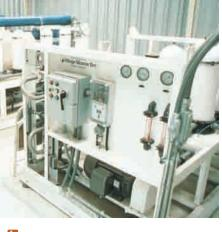
**Figure 11.21** (a) Residents of Catalina Island off the coast of southern California are benefiting from a desalination plant that can supply 132,000 gallons a day, or one-third of the island's daily needs. (b) Machinery in the desalination plant for Catalina Island.
